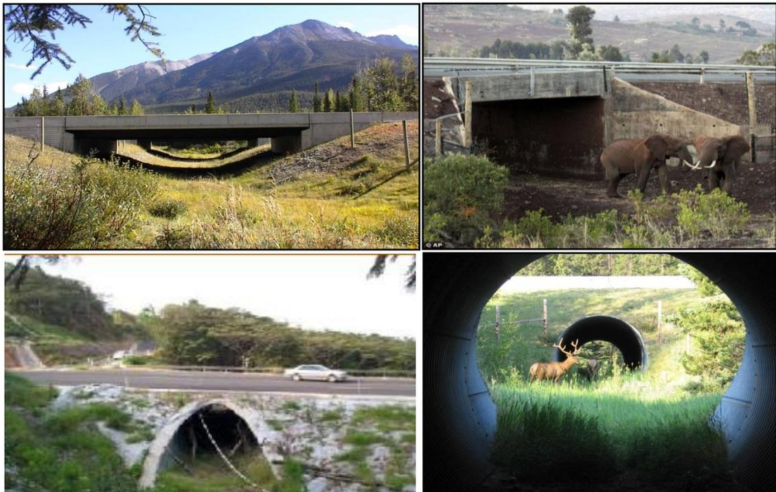
**Figure 5.3: Bridge underpasses and culverts designed to facilitate animal movement**
